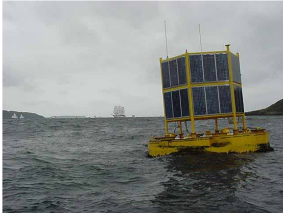
Fig. 6: Coastal Monitoring Station MAREL in the Iroise Sea
